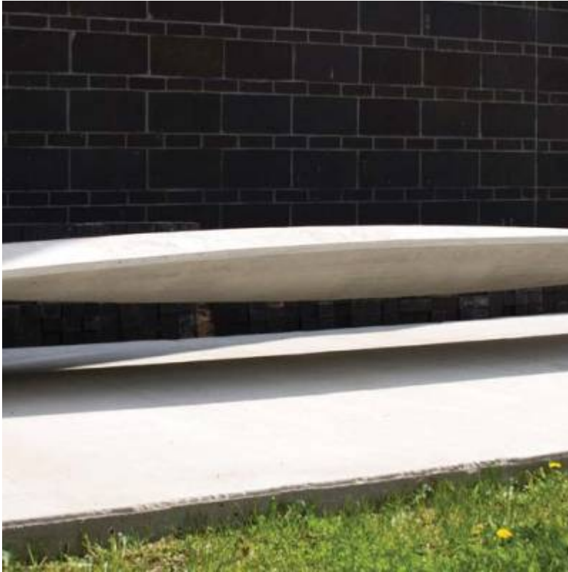
Fig. 41. Completed double-curvature lenticular thin-shell vault.
