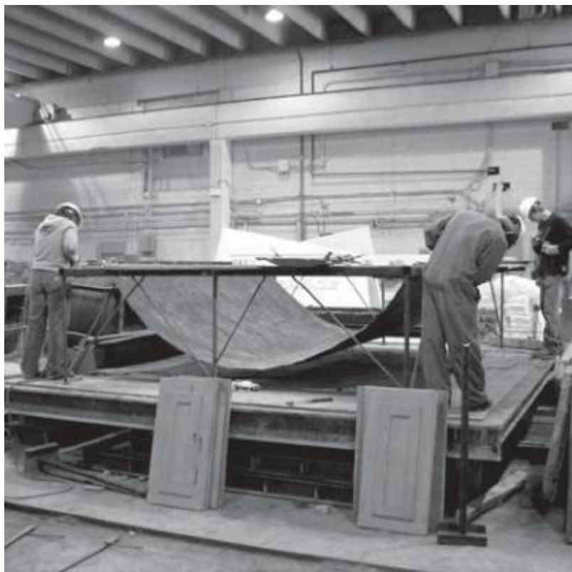
Fig. 22. Step 1 - Geotextile fabric hung from a frame.
