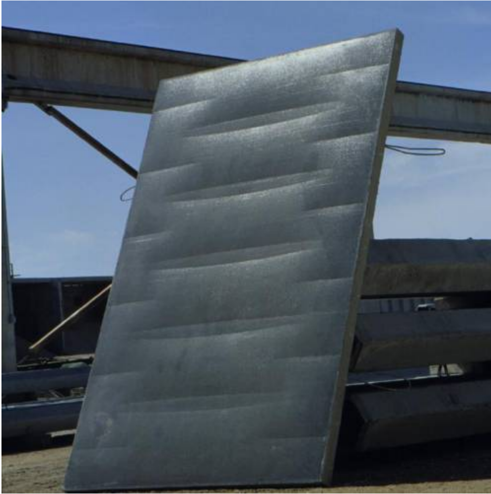
Fig. 10. Completed full scale concrete wall panel.
