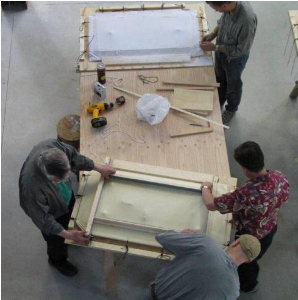
Fig. 2. Model wall panel formwork.
