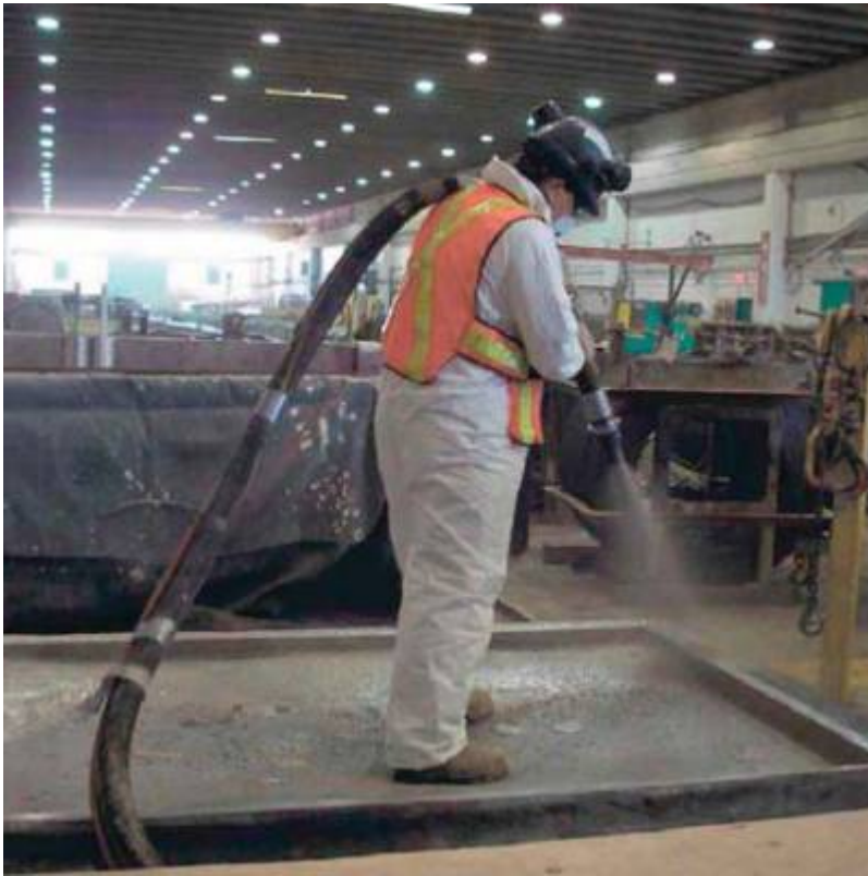
Fig. 28. A uniform thickness of fiber-reinforced shotcrete is placed over the...
