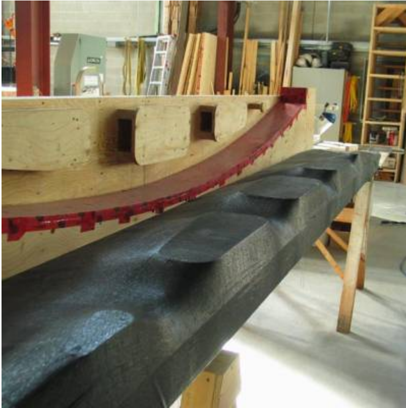
Fig. 3. Model truss formwork.
