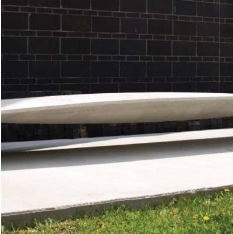
Fig. 41. Completed double-curvature lenticular thin-shell vault.
