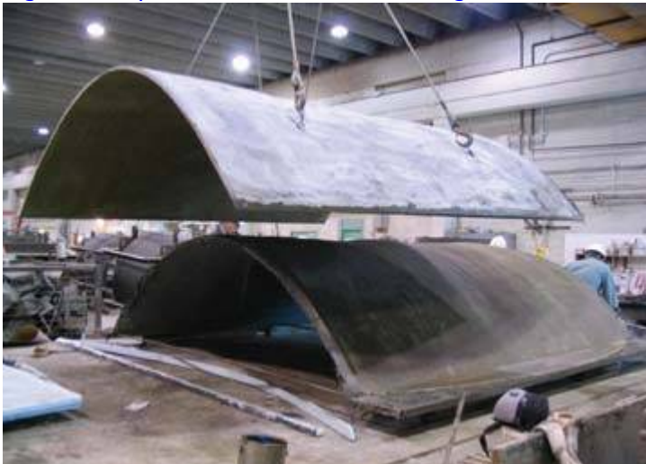
Fig. 23. Step 2- Uniform layer of GFRC is applied.
