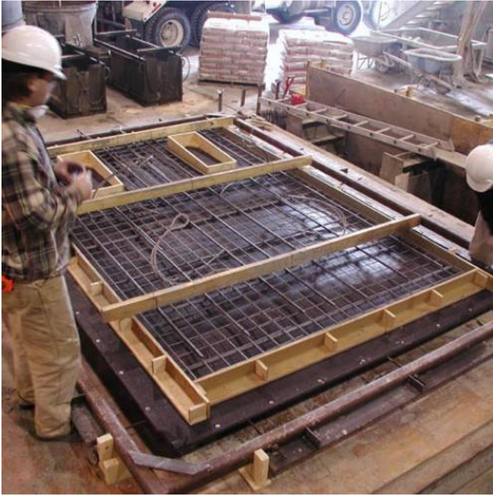
Fig. 5. Securing fabric and placing reinforcement in full scale wall panel...
