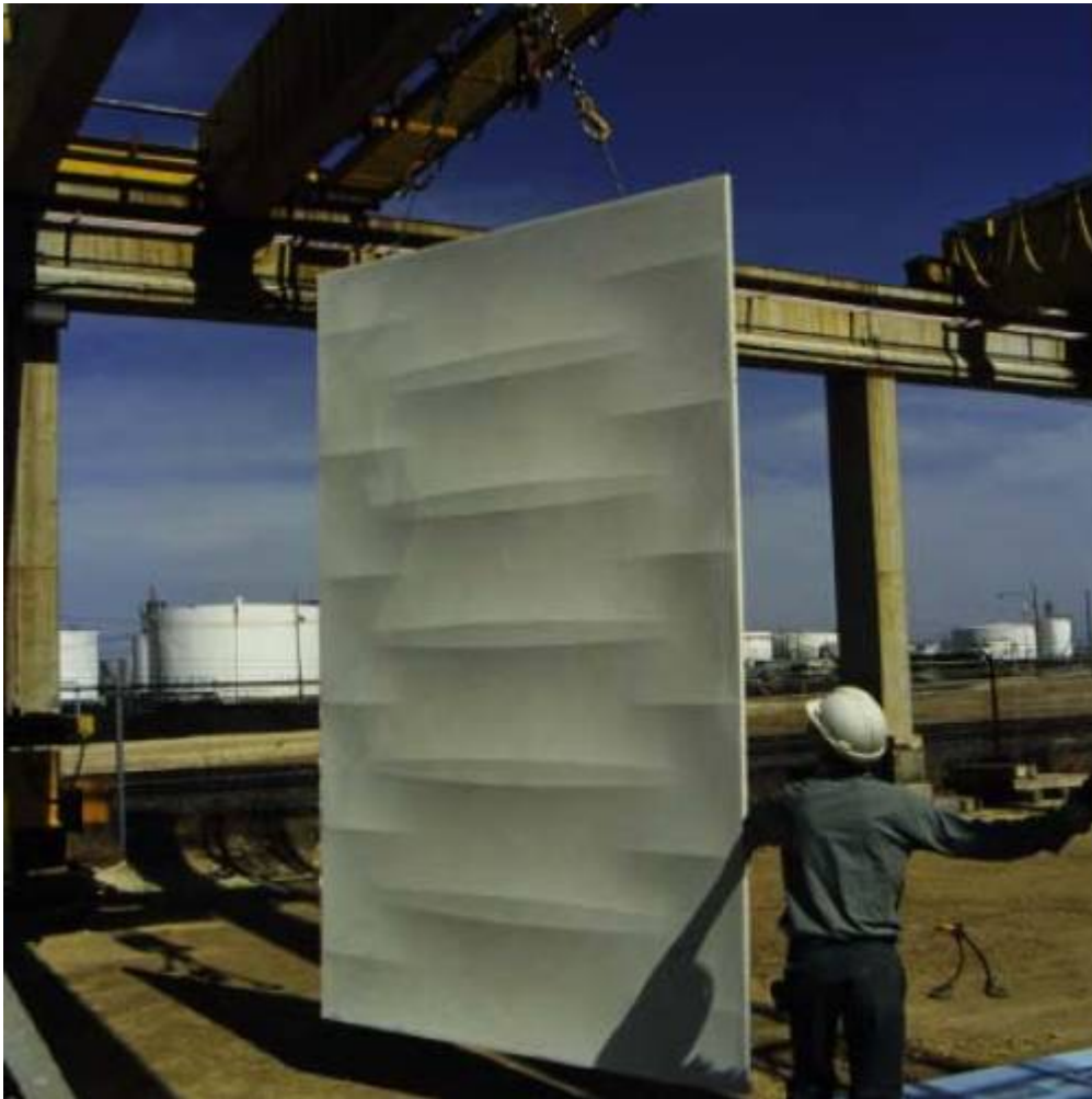
Fig. 11. Completed full scale reverse cast GFRP panel.
