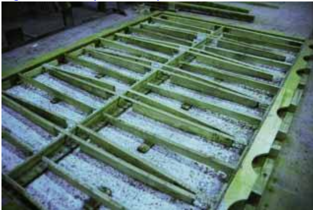
Fig. 9. Formwork for full scale wall panel.
