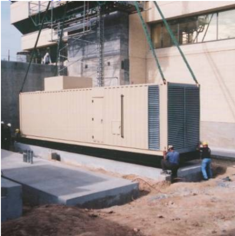
Fig. 5. Setting generators.
