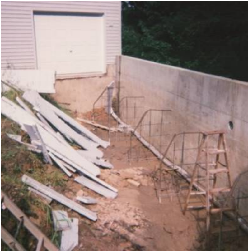
Retaining Wall Repair
