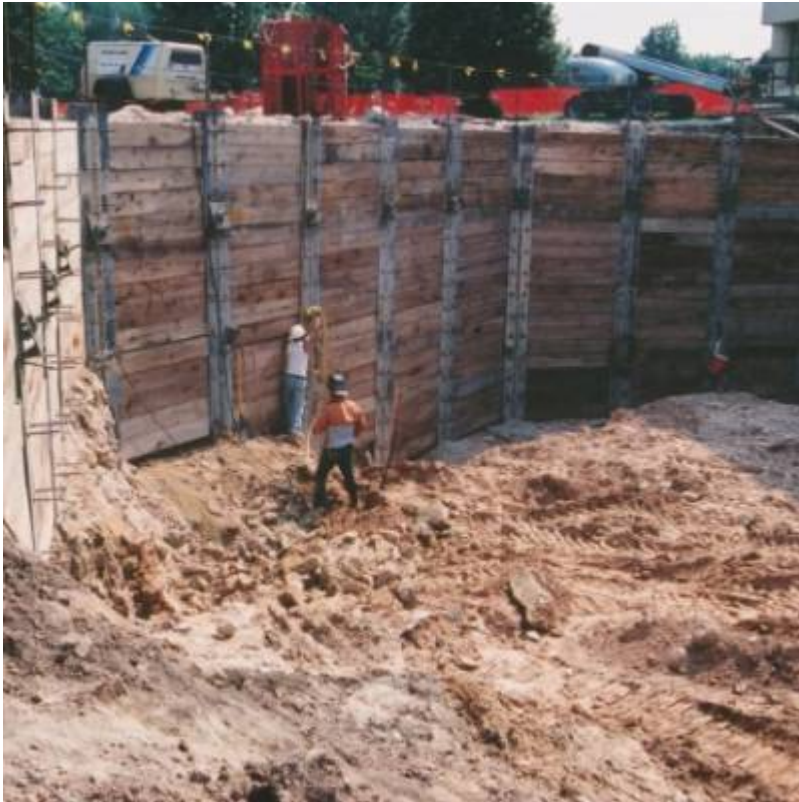
Fig. 1. Excavation and soldier beam earth retention system.
