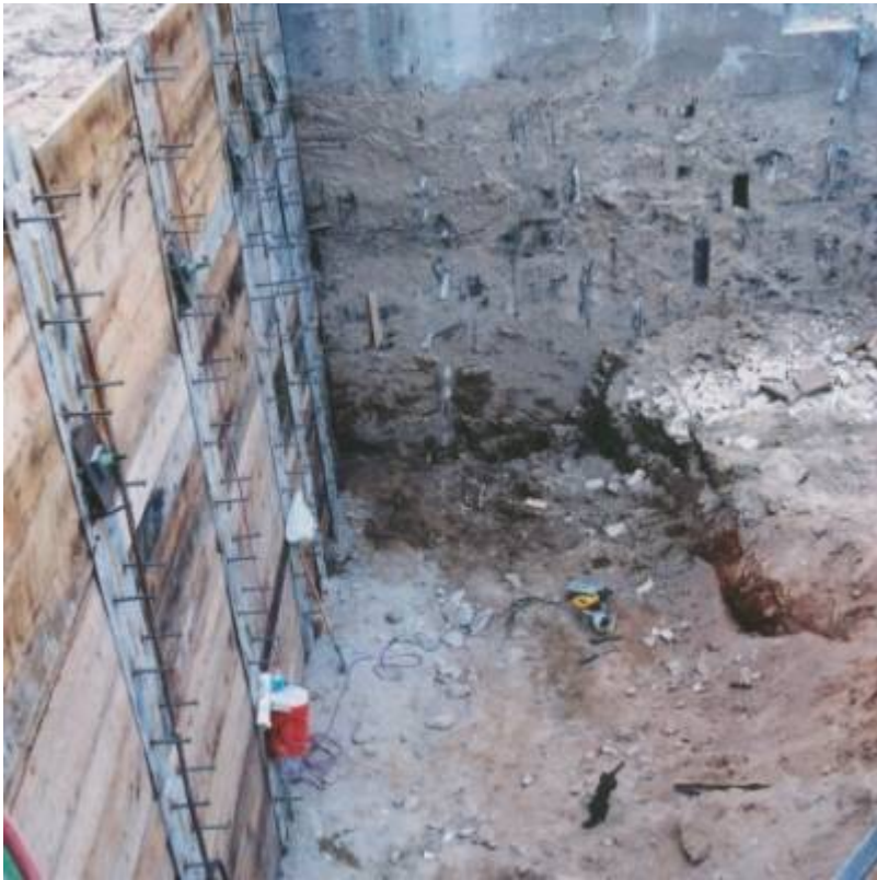
Fig. 2. Excavation and soldier beam earth retention system.
