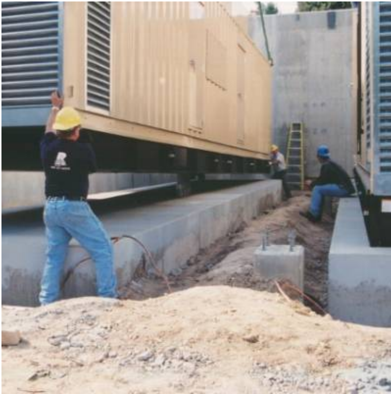
Fig. 4. Setting generators.
