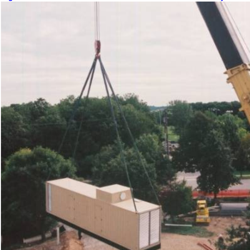
Fig. 3. Setting generators.
