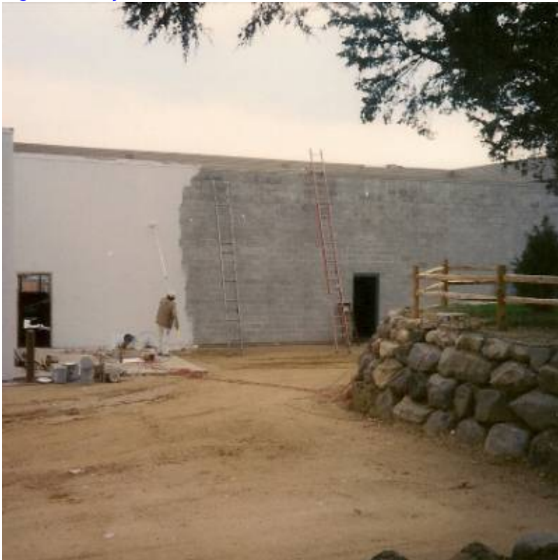
Fig. 6. Sunnyside Retail Center.
