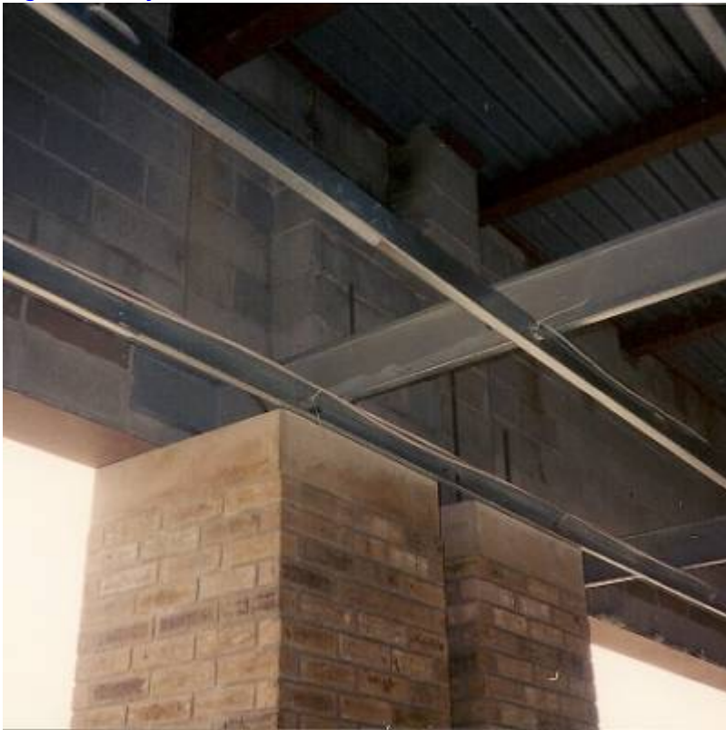
Fig. 4. Sunnyside Retail Center.
