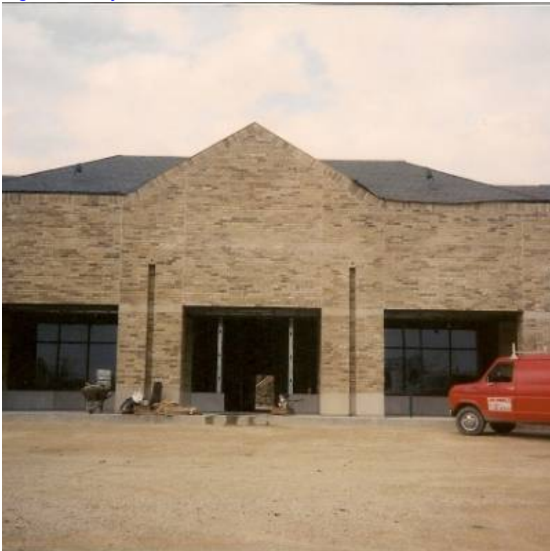
Fig. 2. Sunnyside Retail Center.
