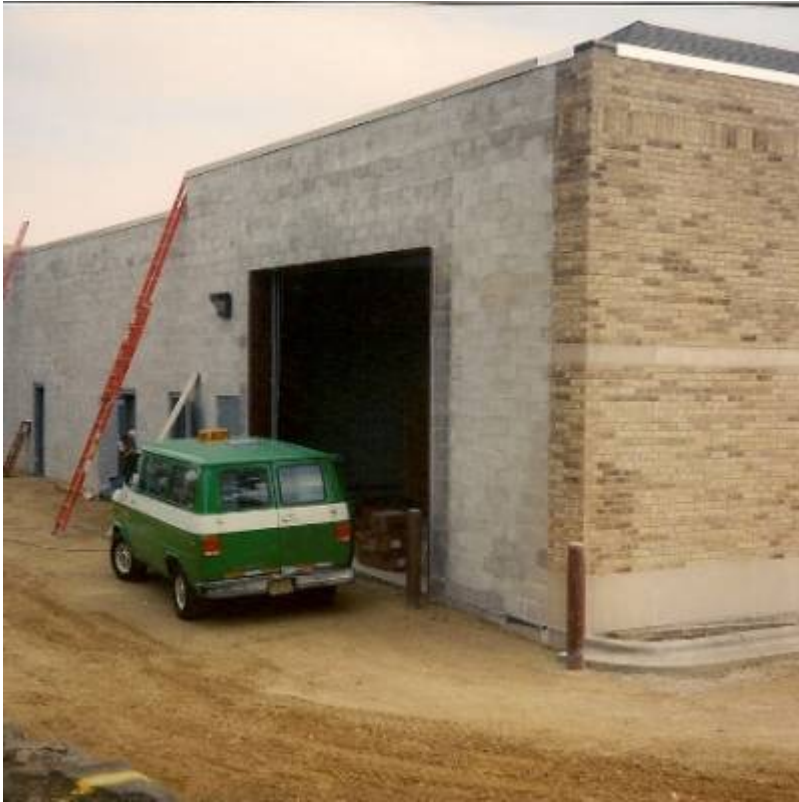
Fig. 5. Sunnyside Retail Center.
