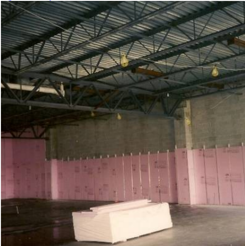
Fig. 8. Sunnyside Retail Center.
