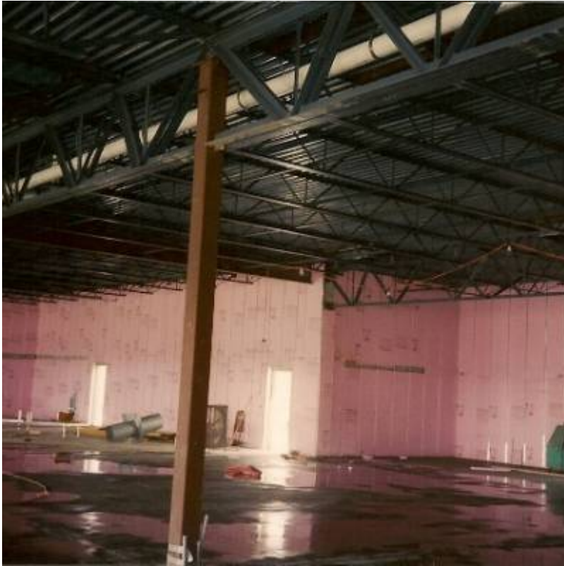
Fig. 7. Sunnyside Retail Center.
