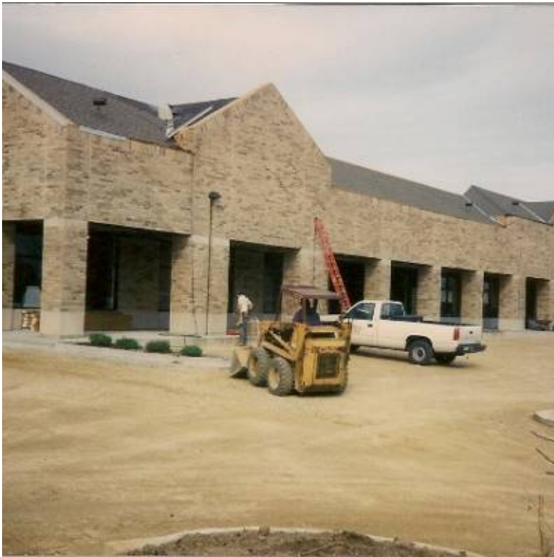
Fig. 1. Sunnyside Retail Center.
