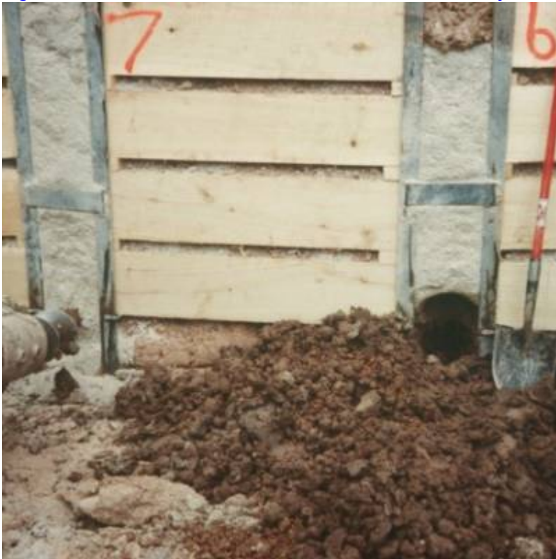
Fig. 5. Installation of soldier beam earth retention system.
