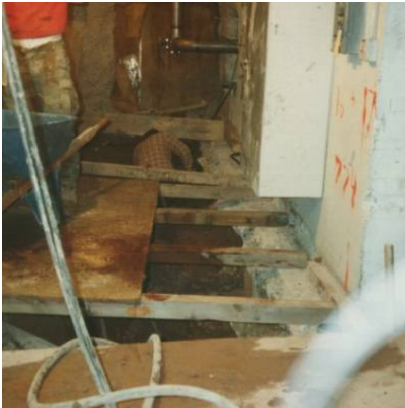
Fig. 8. Underpinning existing foundations.
