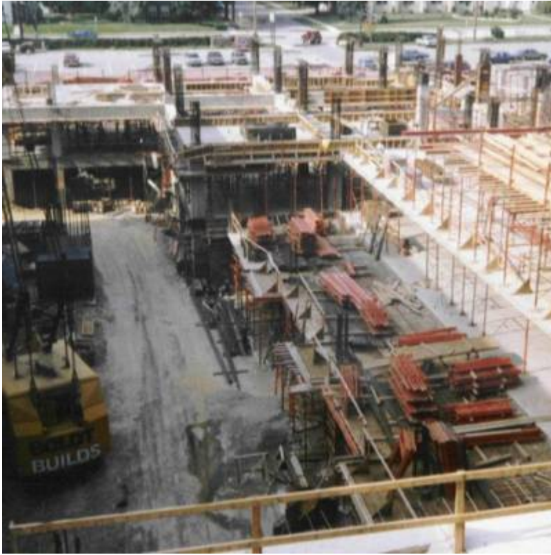
Fig. 24. Concrete framing systems - beam and slab and flat slab with drops.
