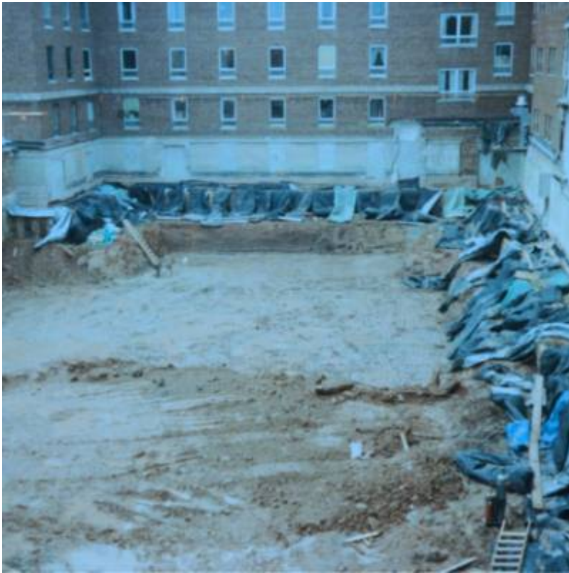
Fig. 2. Start of excavation.
