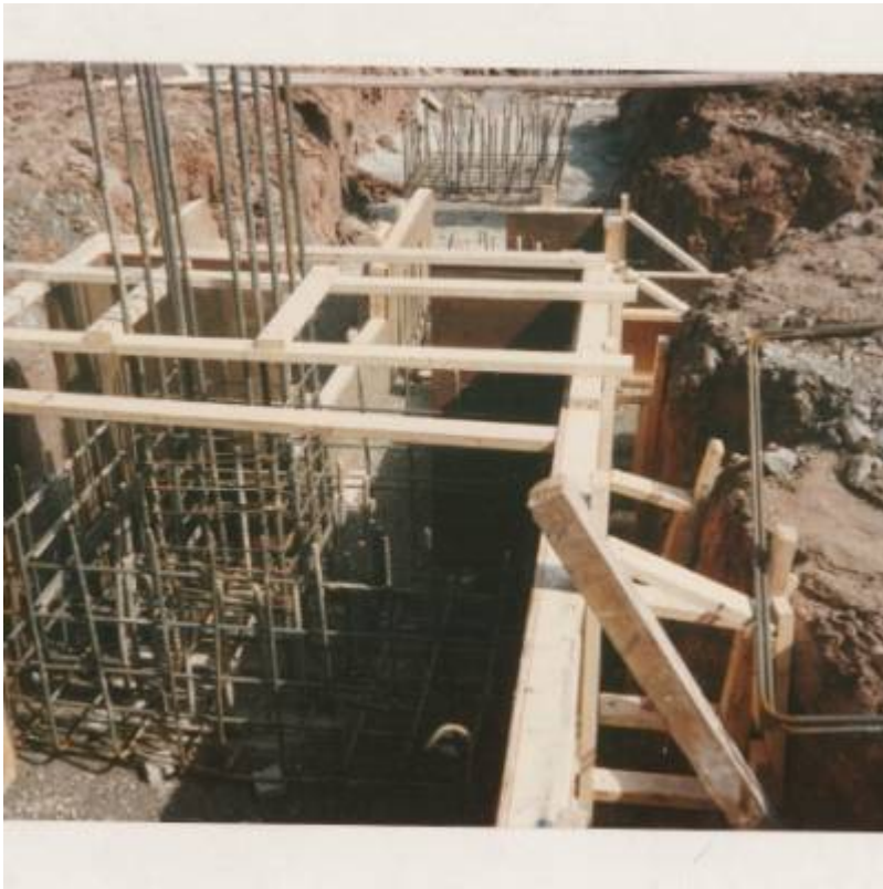
Fig. 18. Foundations - pier caps and grade beams.
