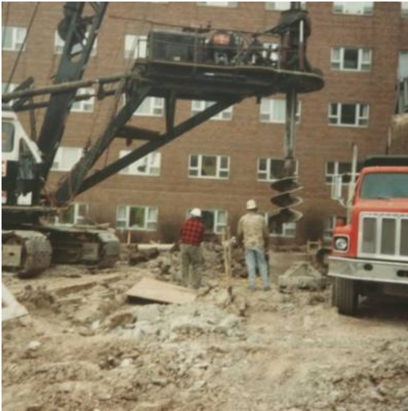
Fig. 12. Drilled pier installation.
