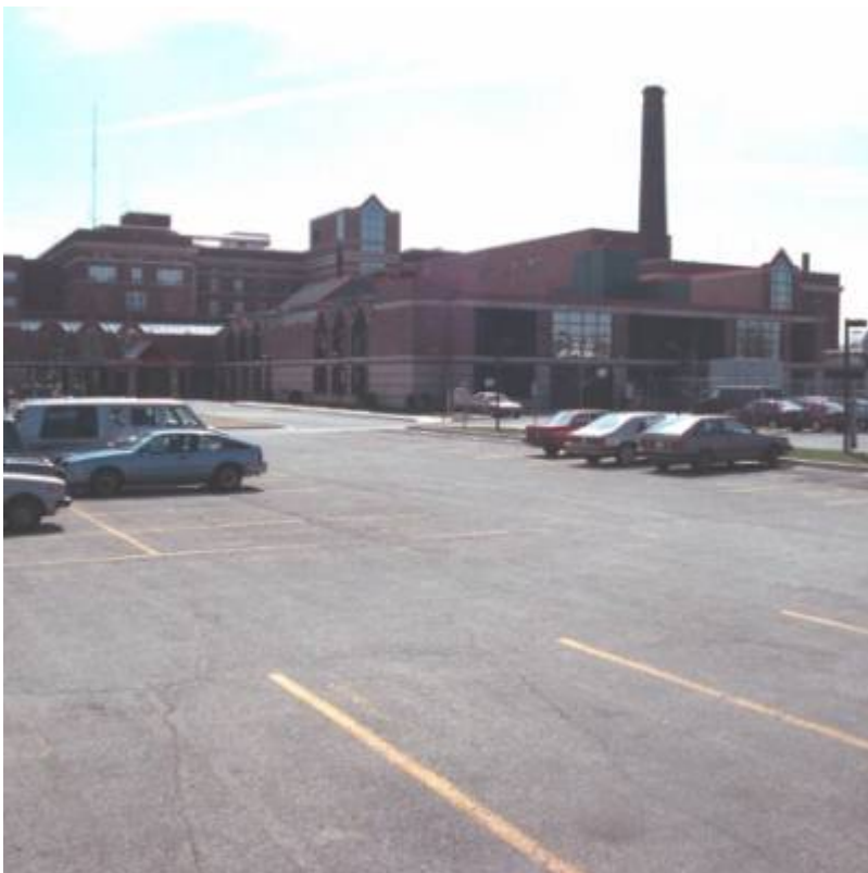
Fig. 25. Emergency entrance and physical plant additions.
