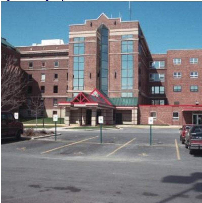
Fig. 27. New main entrance and reception area addition.
