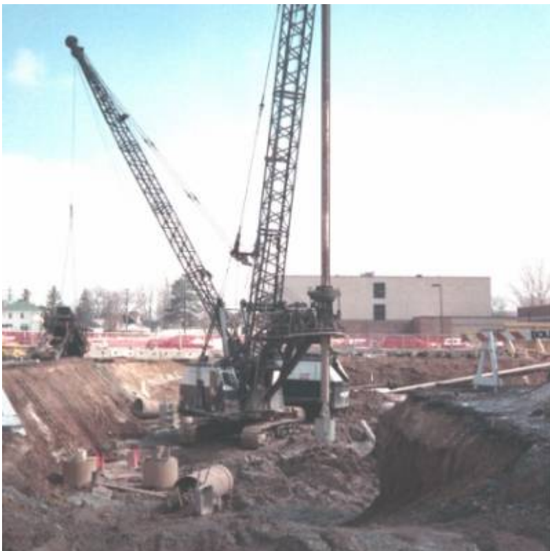
Fig. 11. Deep foundations utilized drilled piers.
