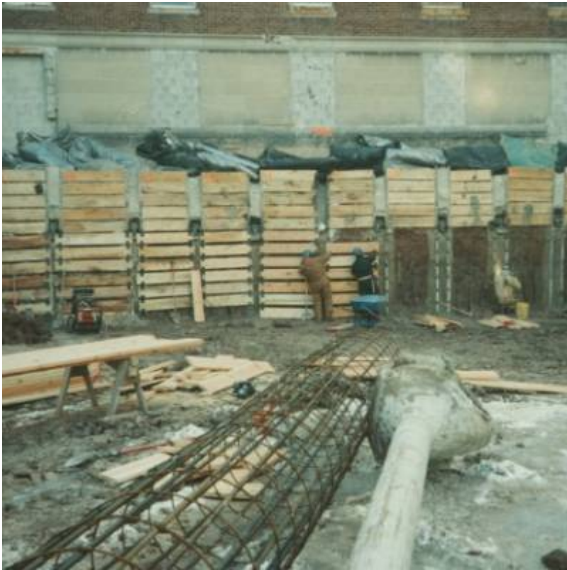
Fig. 4. Excavation and installation of earth retention system.
