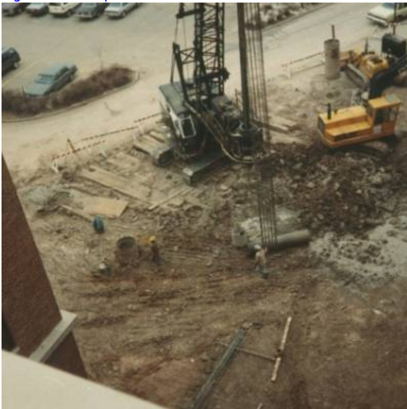
Fig. 13. Setting rebar cage in drilled pier.
