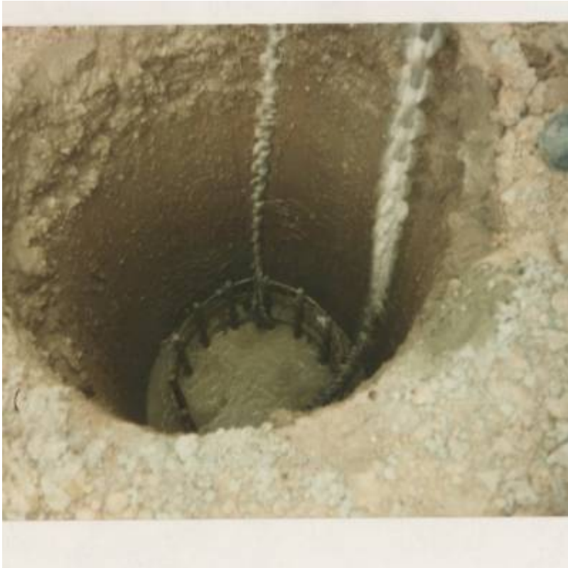
Fig. 15. Drilled pier after concrete has been placed.
