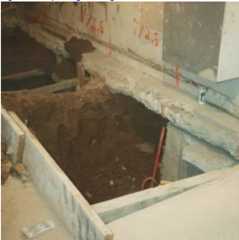
Fig. 8. Underpinning existing foundations.
