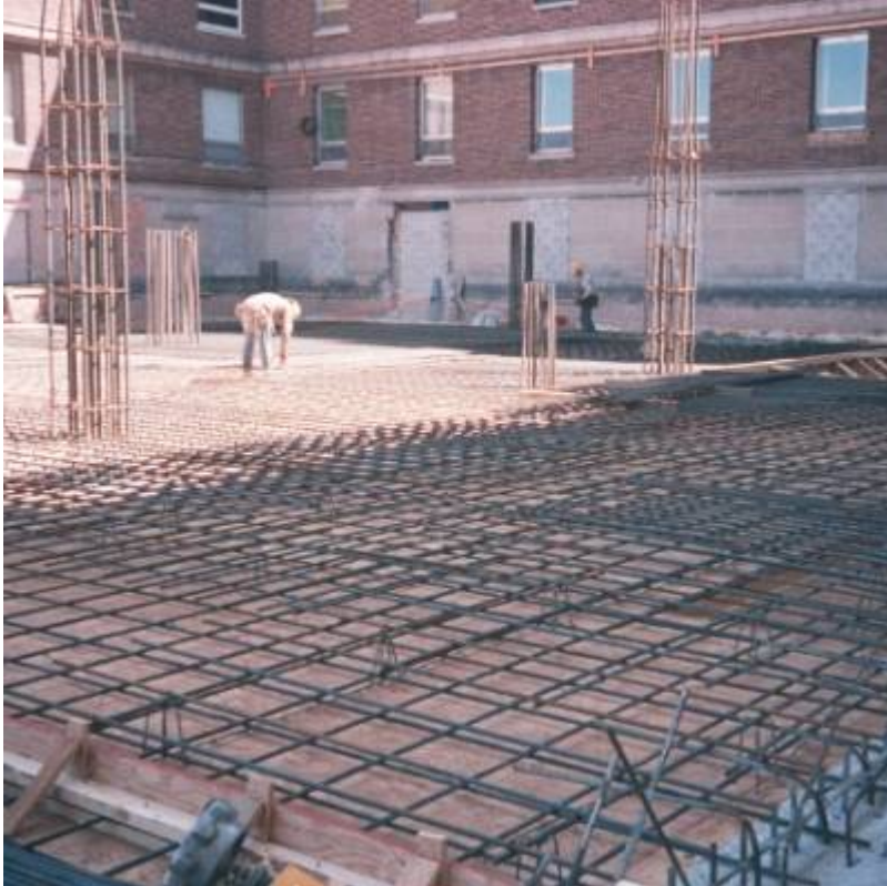
Fig. 22. Floor framing system - flat slab with drops.
