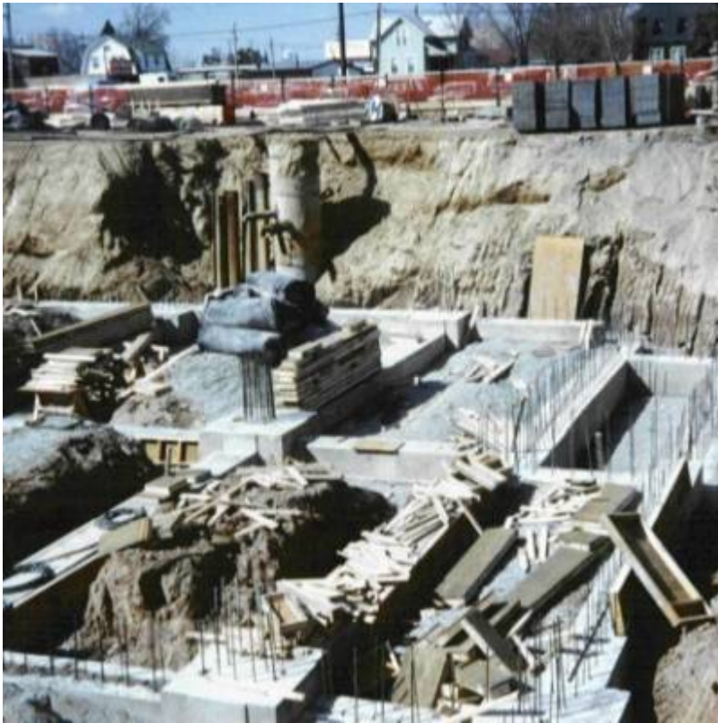
Fig. 20. Foundations - pier caps and grade beams.
