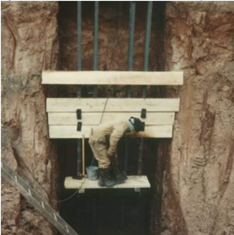
Fig. 7. Underpinning existing foundations.
