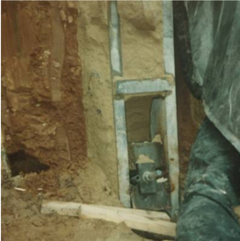
Fig. 6. Installation of soldier beam earth retention system.
