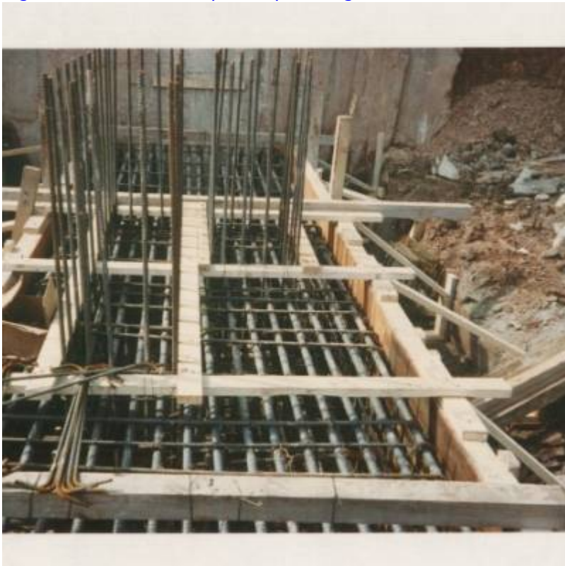
Fig. 19. Foundations - pier caps and grade beams.
