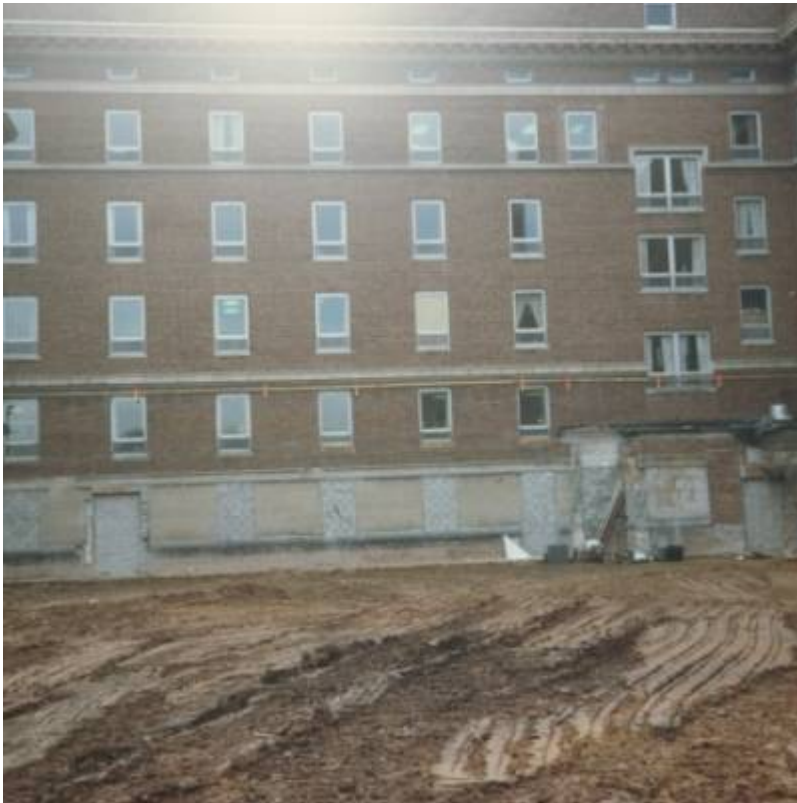
Fig. 1. Site prepped for excavation after demolition of previous structures.
