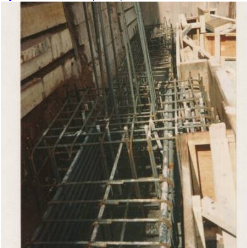
Fig. 17. Foundations - pier caps and grade beams.
