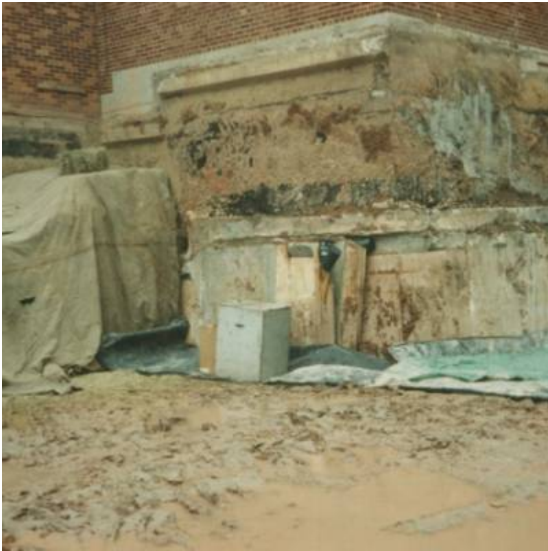
Fig. 9. Underpinning foundations for existing hospital pool.
