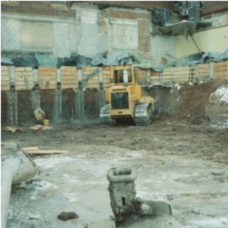
Fig. 3. Excavation and installation of earth retention system.
