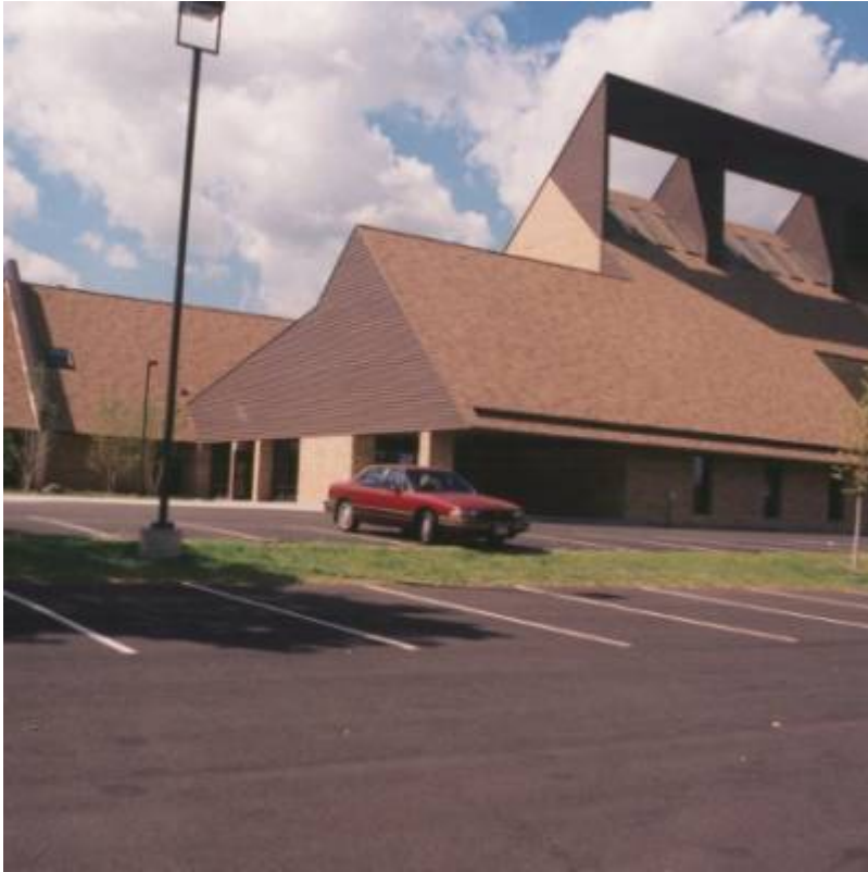
Fig. 4. St. Thomas Aquinas church and school addition.
