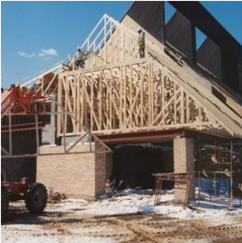
Fig. 2. St. Thomas Aquinas church and school addition.
