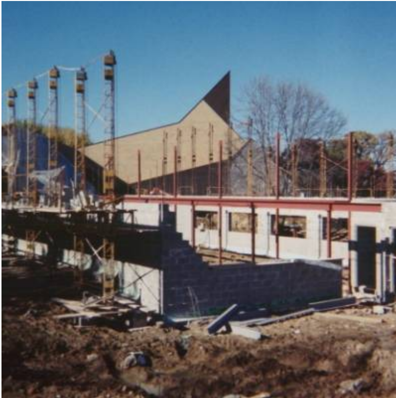
Fig. 1. St. Thomas Aquinas church and school addition.
