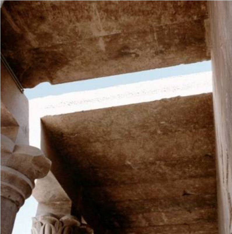
Fig. 5. Roof detail eastern colonnade.
