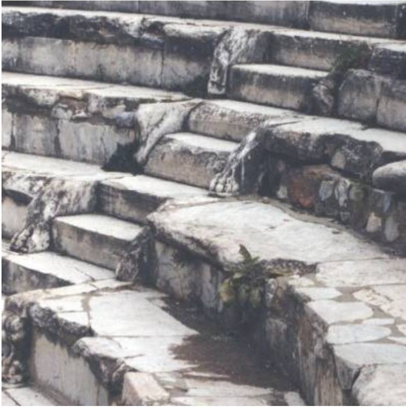
Fig. 5. The Odeion, noted detail at stairs.
