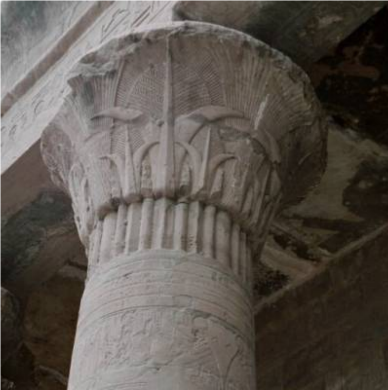
Fig. 6. Column capital detail from peristyle court.
