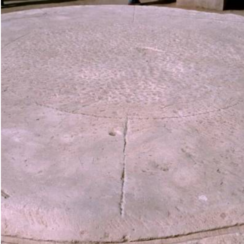
Fig. 1 Column base showing masons guide lines.
