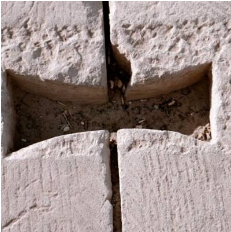
Fig. 11. Dovetail slot in wall of Kom-Ombo Temple.
