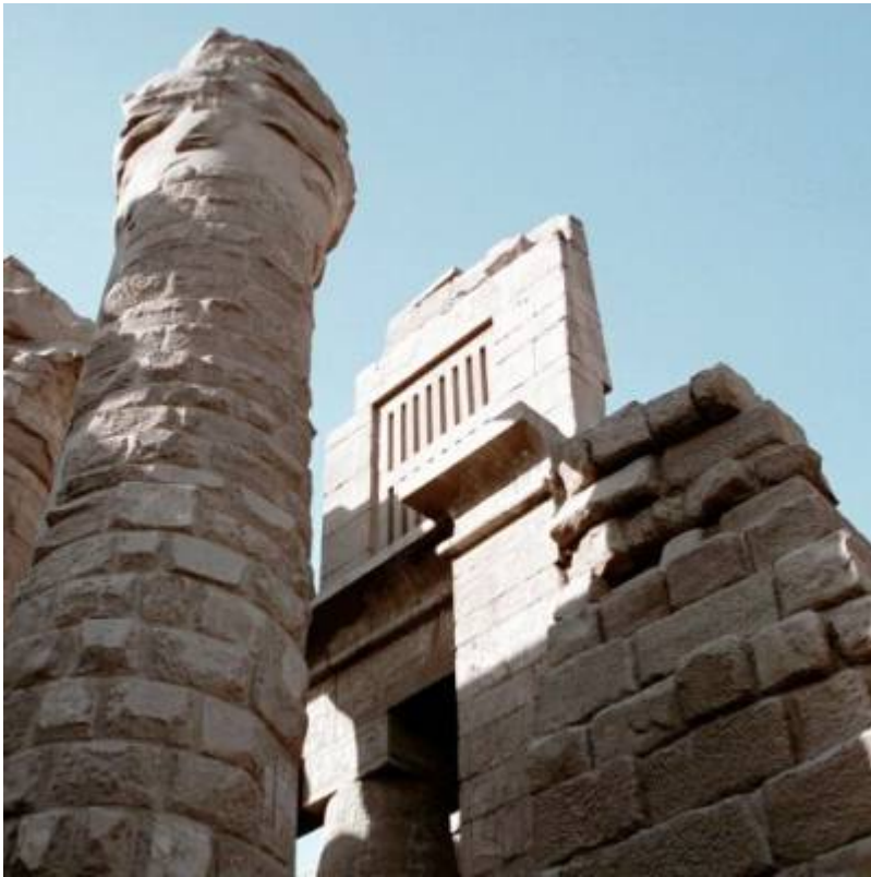
Fig. 11. Unfinished column and wall.
