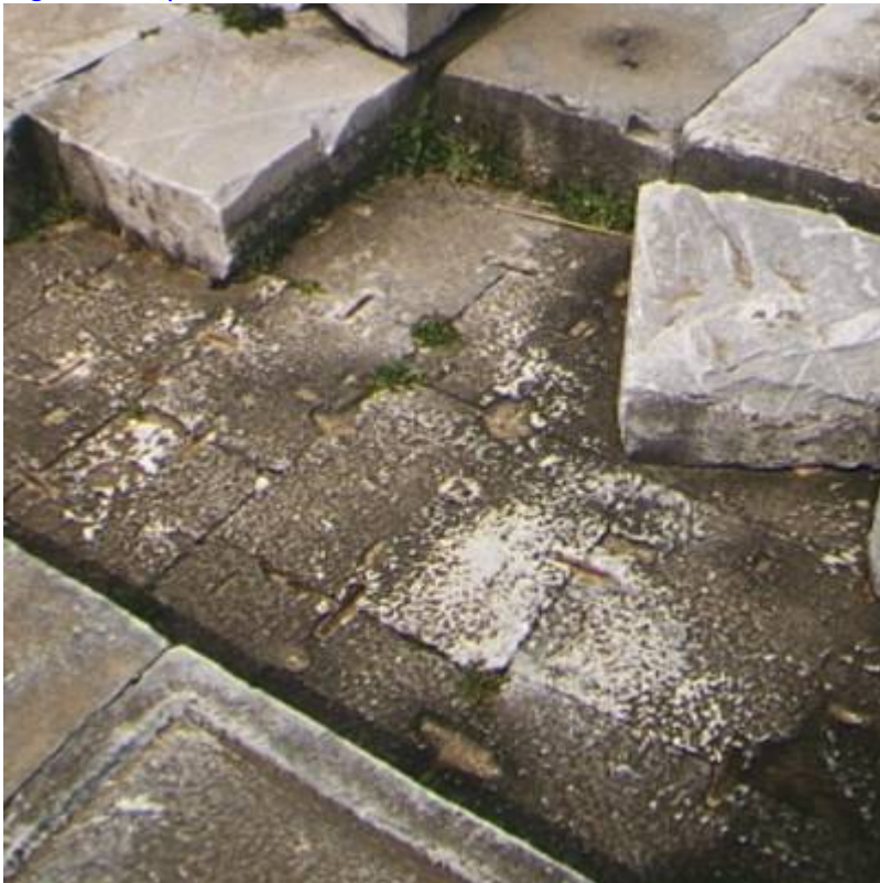
Fig. 8. Temple of Athena, paving anchor detail.
