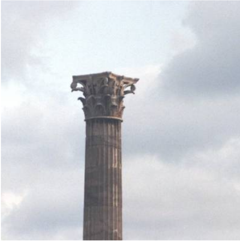
Fig. 3. Corinthian column detail.
