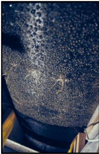
Fig. 12. Filtration of excess water and air bubbles through geotextile fabric (C.A.S.T. photo).
