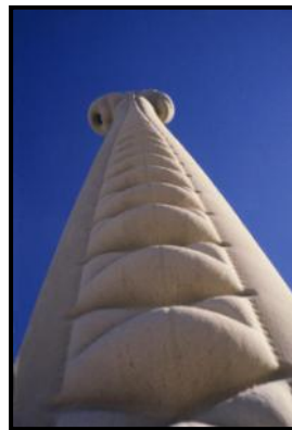
Fig. 17. Completed full-scale column (C.A.S.T. photo).
