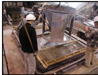
Fig. 10. Placing concrete in full-scale wall panel formwork (C.A.S.T. photo).
