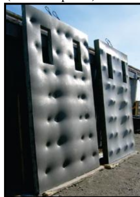
Fig. 11. Completed concrete wall panels (C.A.S.T. photo).
