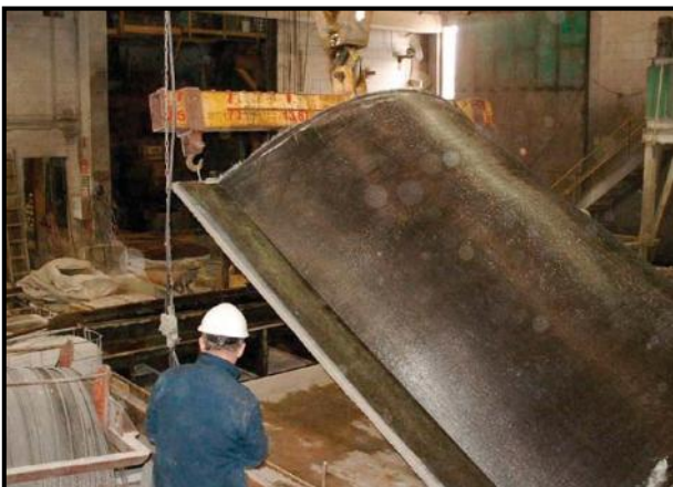
Fig. 20. Step 3 – Resulting funicular shell is inverted to form mold (C.A.S.T. photo).
