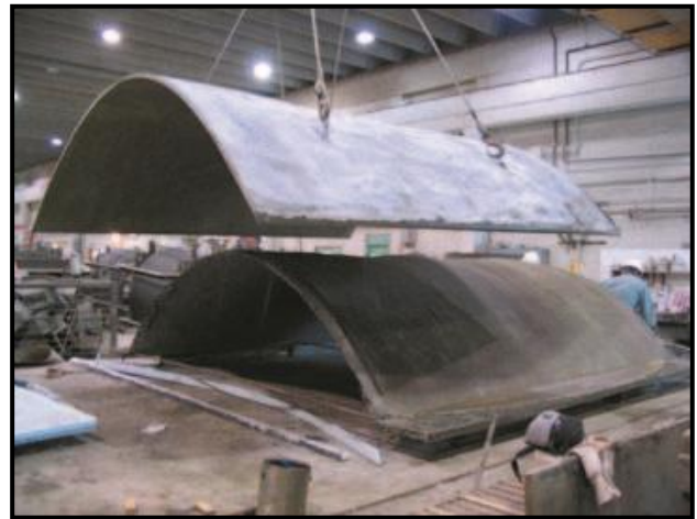
Fig. 21. Step 4 – Thin-shell funicular GFRC vault produced from mold (C.A.S.T. photo).
