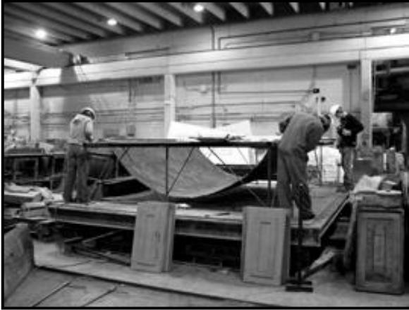
Fig. 18. Step 1 – Geotextile fabric hung from a frame (C.A.S.T. photo).
