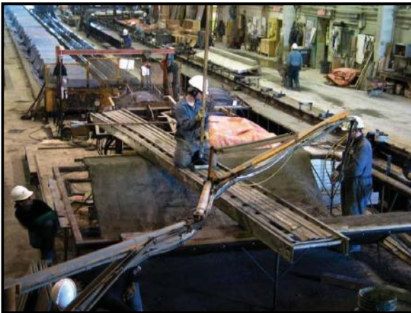
Fig. 19. Step 2- Uniform layer of GFRC is applied (C.A.S.T. photo).
