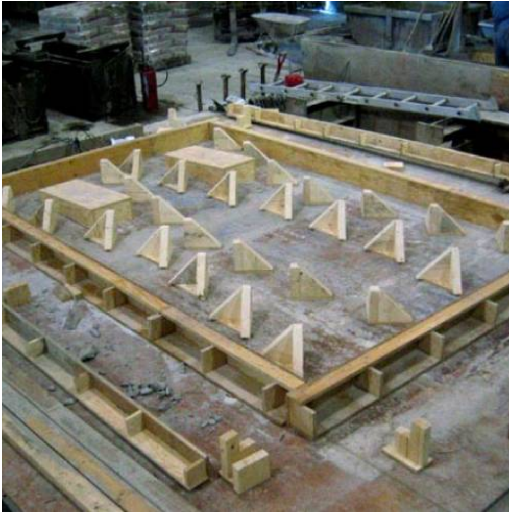
Fig. 4. Placing blockouts and interior supports prior to stretching in fabric in...
