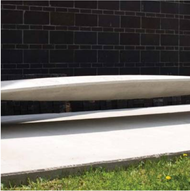
Fig. 41. Completed double-curvature lenticular thin-shell vault.
