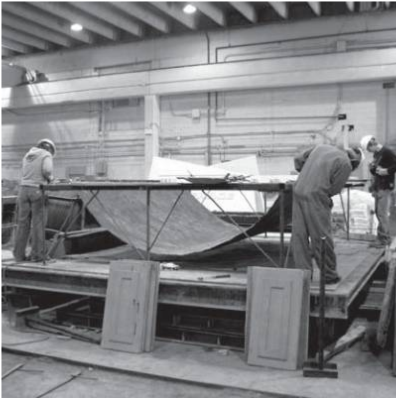
Fig. 22. Step 1 - Geotextile fabric hung from a frame.
